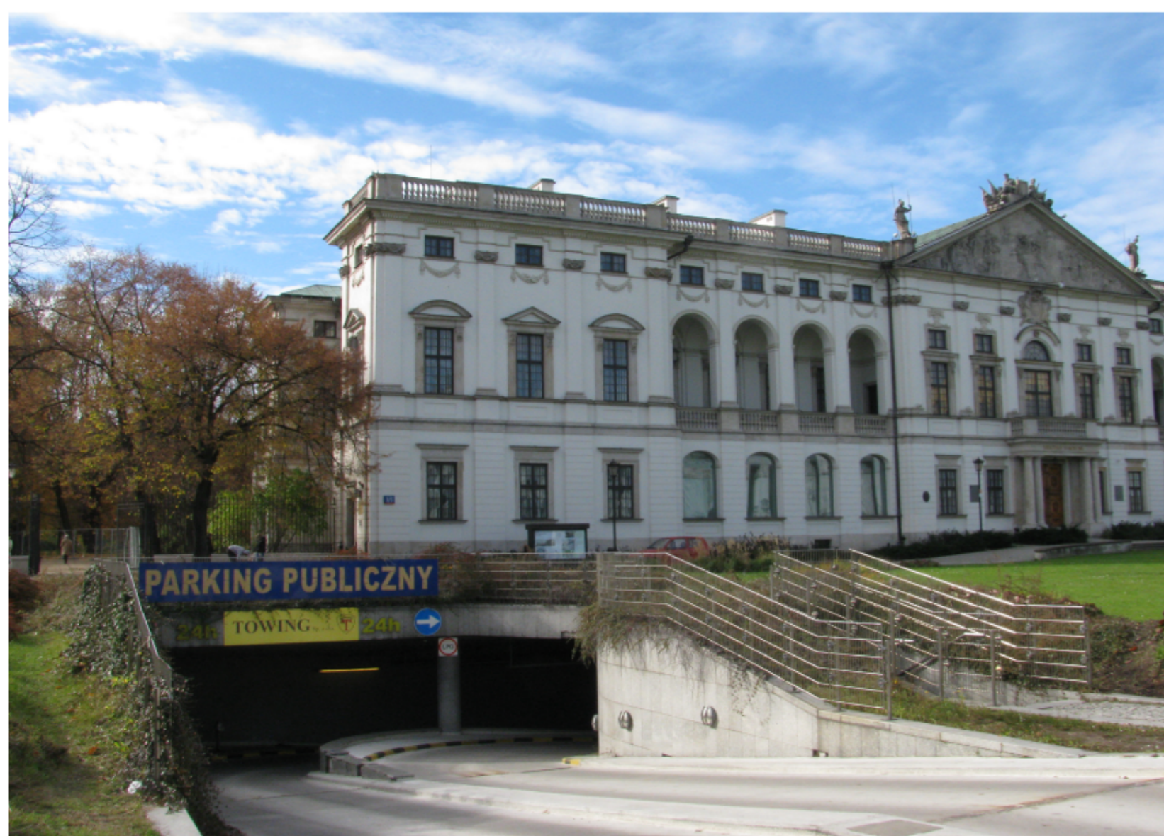
The view of the north east elevation of the Krasinski Palace. The new public parking under the Krasinski Square causes the permanent water activity on the foundations of the Palace. The Palace has two axes of symmetry, except for the roof - there is a walking terrace on the north-east side. That is where the leak may have started.
